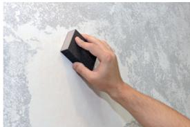
Clean the wall using emery and high grade sand paper/putty blade/wire brush to remove loose particles, sand, dust, lubricants etc.
