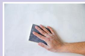
Scrub the wall with suitable emery paper to remove the marks of blade if needed.
