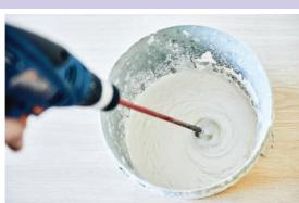
Mix the putty and water thoroughly with putty mixing machine. Leave it for 5-10 minutes and re-stir for getting homogenous paste.
