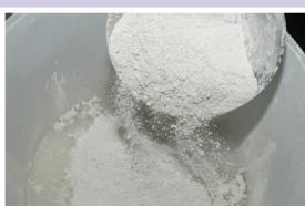
Prepare the putty paste by adding 35-40% clean water to Assure Mix Wall putty (350-400ml/Kg of putty).
