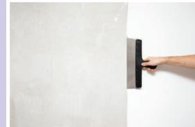
Apply the first coat of wall putty with the help of putty blade and let it dry for at least 4-6 hours or as per the site condition.
